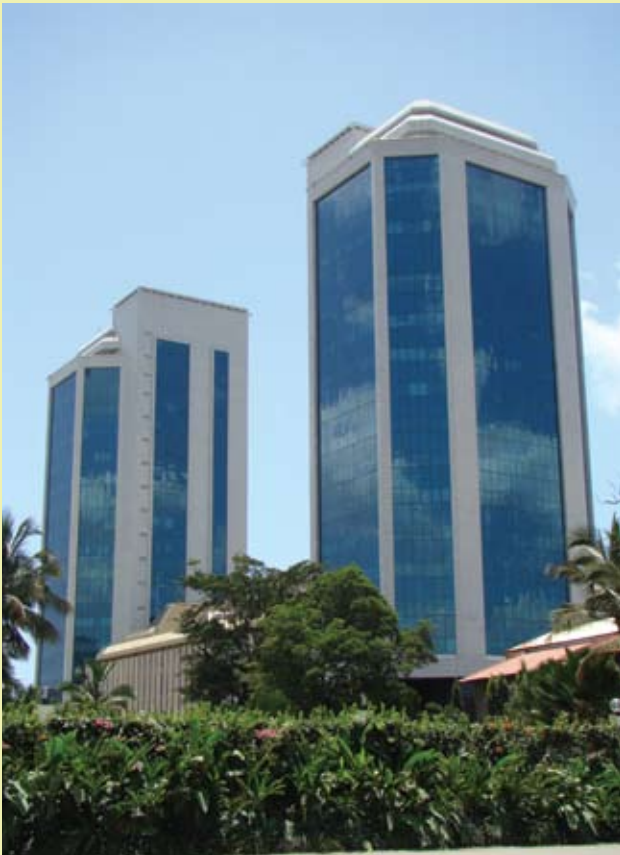
Twin Towers which house the Headquarters of Bank of Tanzania responsible to oversee the development of banking sector in the country.
